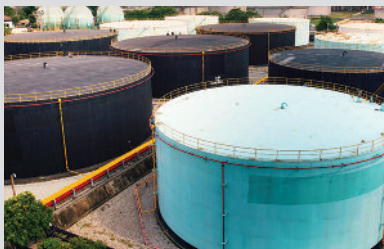
Storage Tank Maintenance
